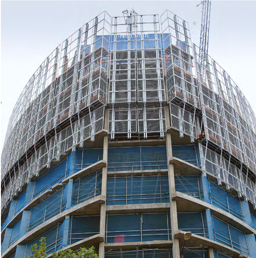
► Complex architecture easily accommodated
