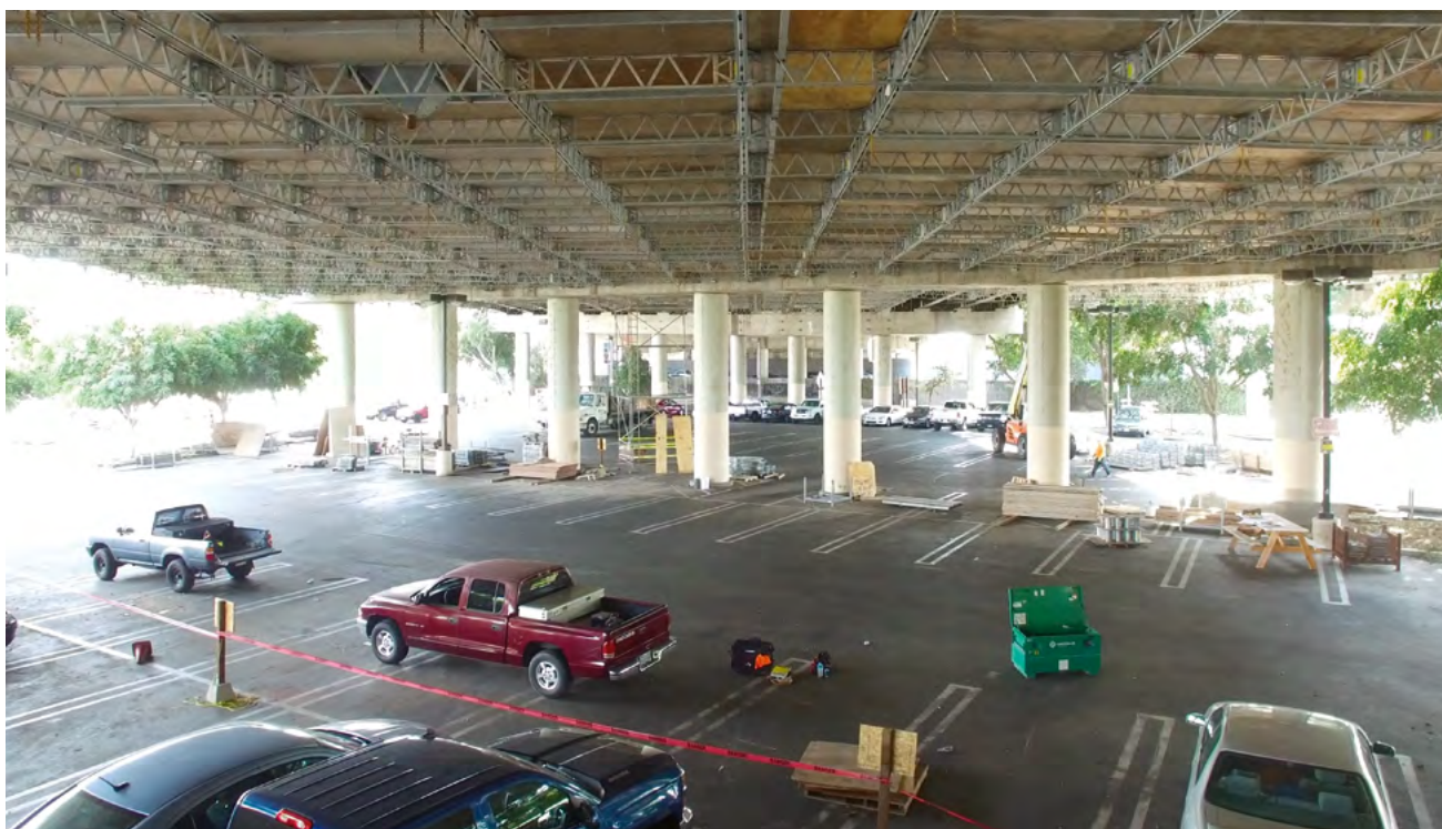
► The QuikDeck suspended platform enables work without interruption, e.g. during bridge renovations. There is usually no need for traffic closures – on or under bridges.
