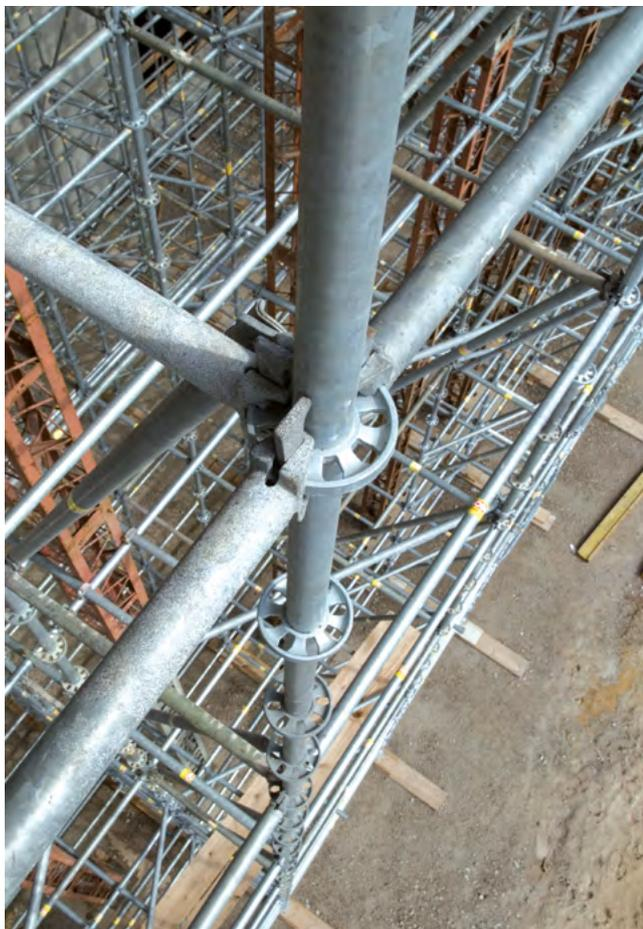
◀ Ideal flexibility as a result of 8 possible connections in horizontal, vertical, and diagonal directions
