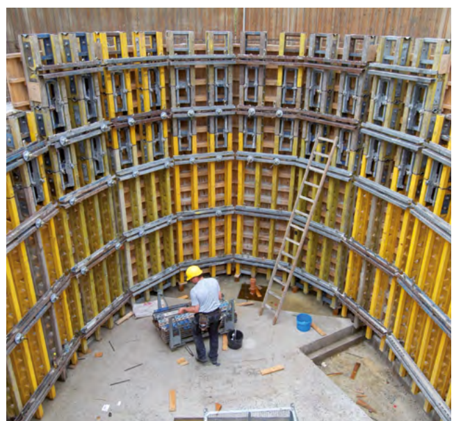
► Desired element heights can be easily attained according to the architectural concrete requirements
