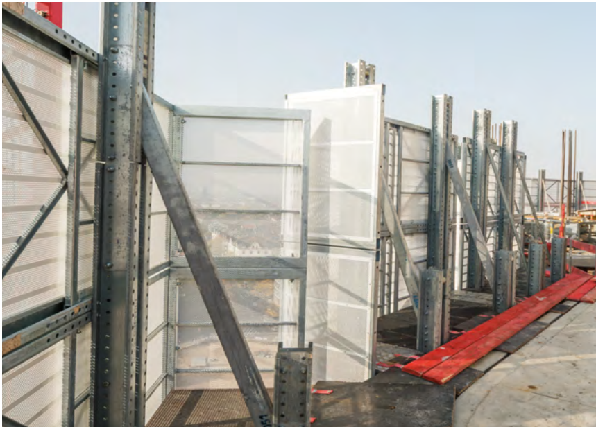
► Improved on-site and public safety due to full enclosure of the working environment
