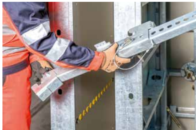
► Formwork clamp for highly tensile and pressure-resistant stop-ends with only one part
