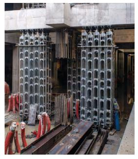
▶ Very high load capacity of up to 210 kN even with small base dimensions of only 25 x 25 cm
